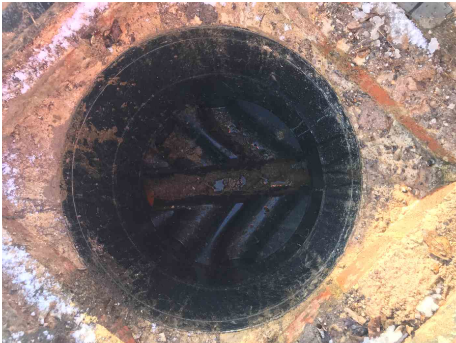
FW0_297b88ea-c95f-4ade-adf3-e6fe0aa89a06_20210125_154111.jpg, 0.00 m General photograph taken at this point at 12 o'clock, internal condition photograph
