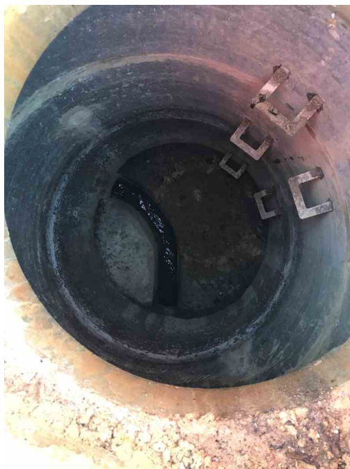
FW1_54342b58-cce7-49af-b937-ccb06922d291_20210125_160054.jpg, 0.00 m General photograph taken at this point at 7 o'clock, internal condition photograph
