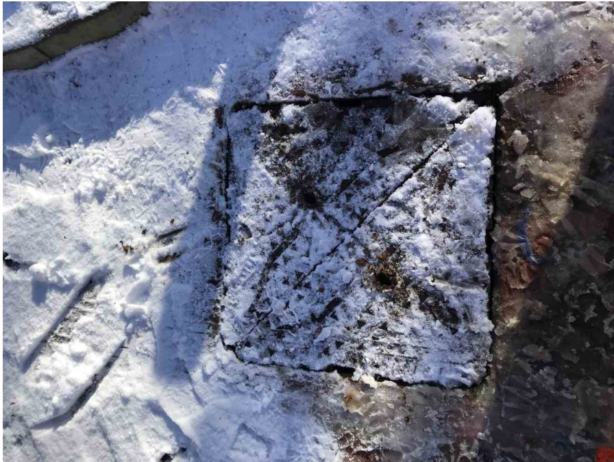
FW0_10975bbc-9b59-4ccc-b3f3-1bc6ccdae2b_20210125_154059.jpg, 0.00 m General photograph taken at this point at 12 o'clock, location photograph
