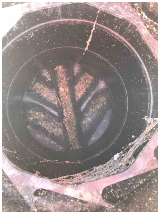
FW4_03b60ff7-6ac0-46c5-8a64-c17bea6da07f_20210125_161137.jpg, 0.00 m General photograph taken at this point at 12 o'clock, internal condition photograph
