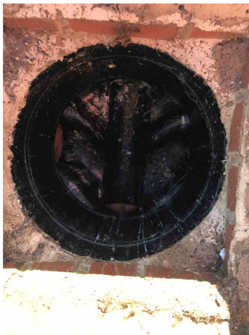
SW1_4f938bc9-7e76-4936-b9f7-40c87d6883d5_20210125_165743.jpg, 0.00 m General photograph taken at this point at 12 o'clock, internal condition photograph
