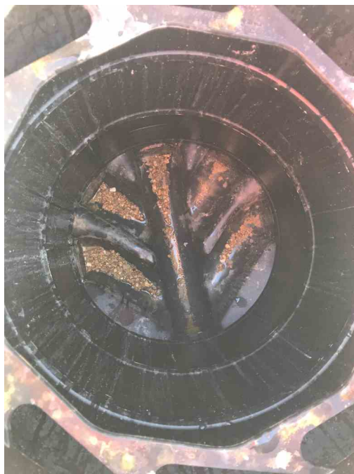
SW0_9cbc04a1-17e6-43a3-a033-5205674992c6_20210125_164809.jpg, 0.00 m General photograph taken at this point at 12 o'clock, internal condition photograph
