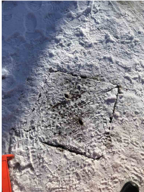
SW1_123ee131-651d-49eb-8f72-47f933e26836_20210125_165724.jpg, 0.00 m General photograph taken at this point at 12 o'clock, location photograph
